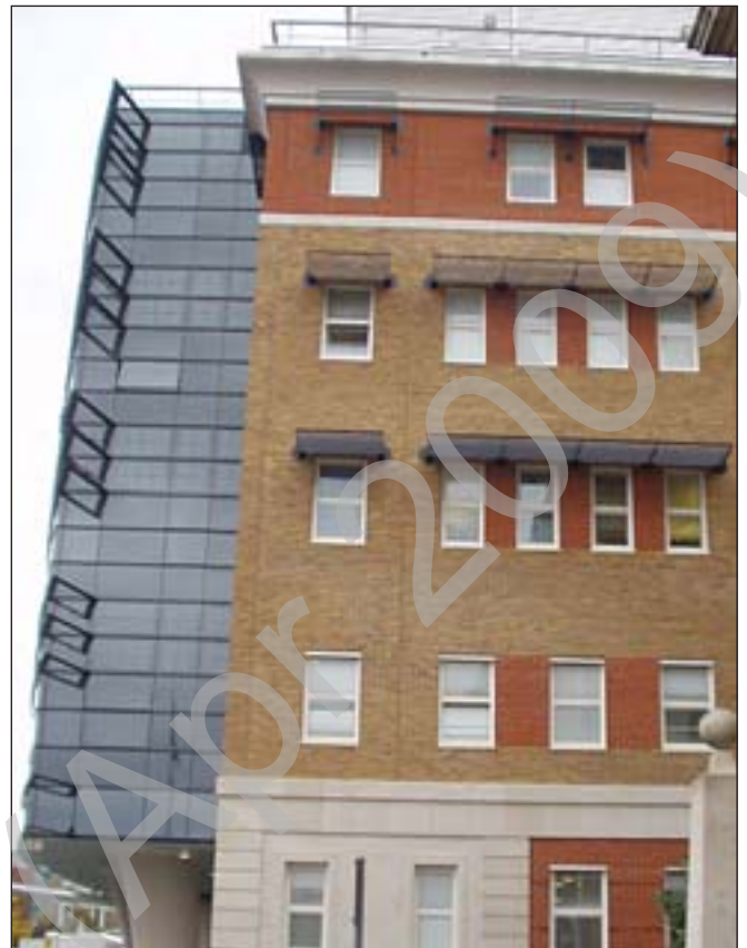
King's College Hospital, London. An external view of the Golden Jubilee Wing at King's College Hospital showing effective window design with external shading to reduce unwanted solar gains
