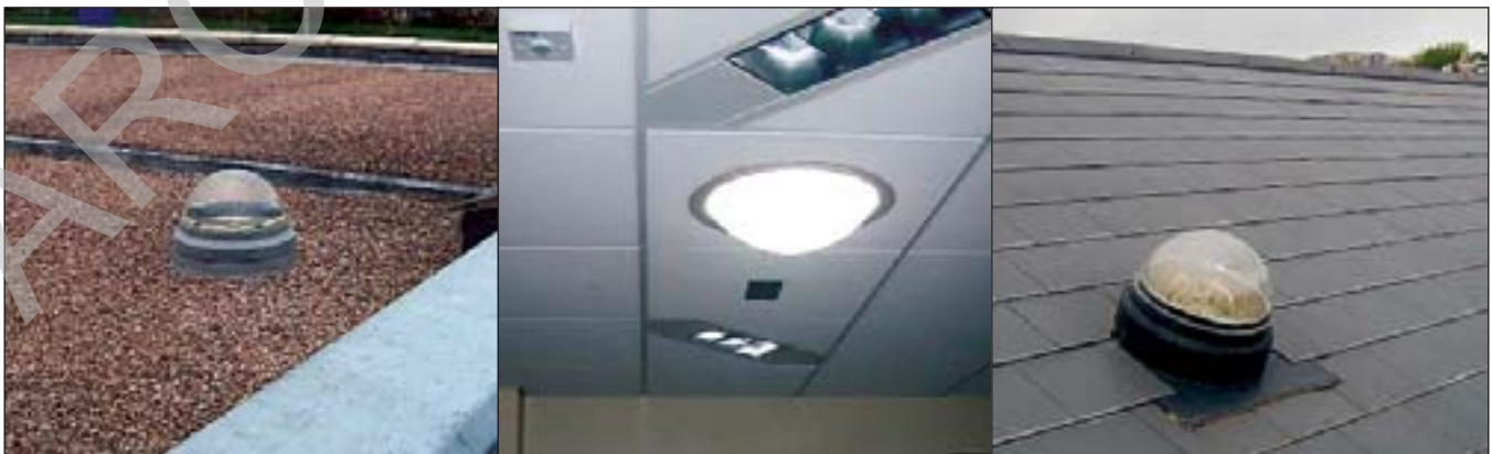
Light pipes have been found to be extremely successful in corridors and deep-plan locations, the purpose being to supplement any artificial lighting with natural light, thus removing the need for lights in the hours of daylight Courtesy of North Devon District Hospital
