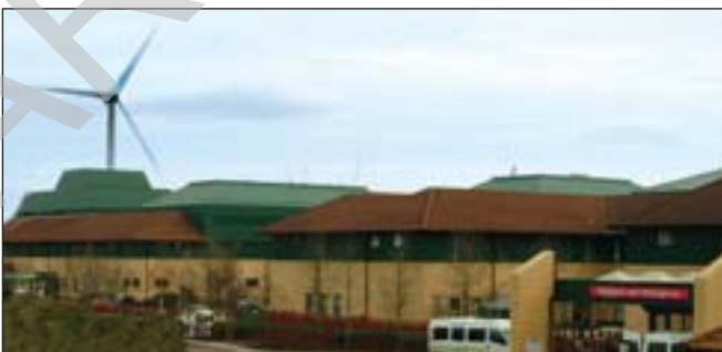
The 660 kW wind turbine at Antrim Area Hospital was the first to be installed on a hospital site in Northern Ireland. The scheme is on track to save £90,000 in its first year of operation.
